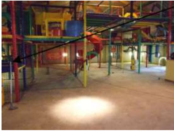
A small area of the soft play area has been coated with waterproof easy clean paint, which needs treatment before drying.
